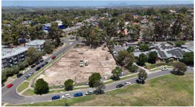
THE NEW UNITS WILL BE SITUATED ON TOWER AVENUE AND BOADLE ROAD, BUNDOORA, ADJACENT TO OUR AGED CARE HOME, WHICH CAN BE SEE AT THE RIGHT OF THE PHOTO ABOVE.
